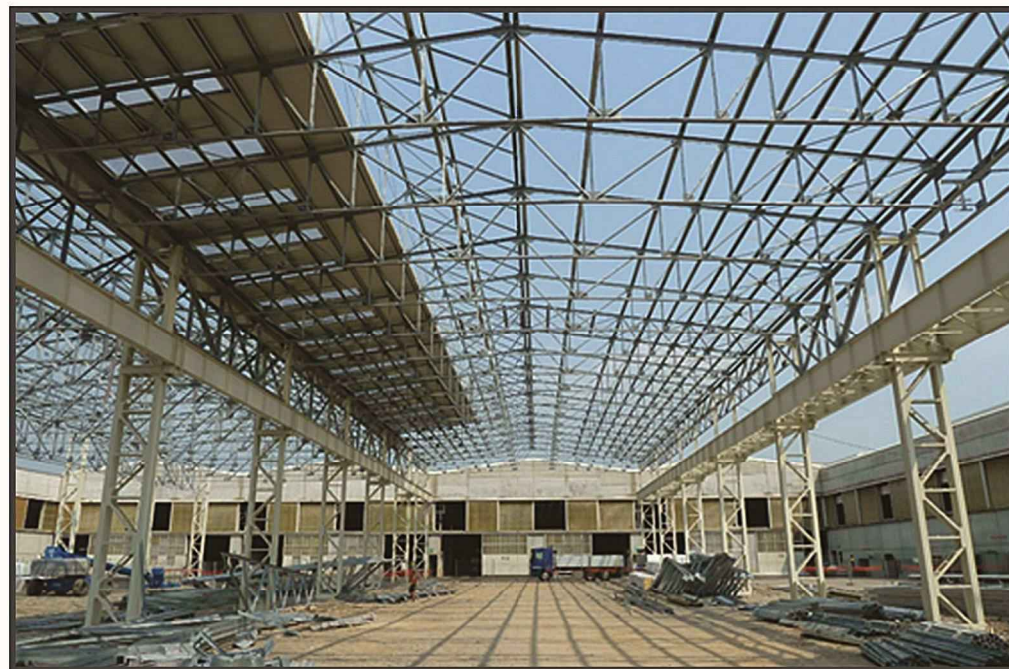
2009: 15.000 m2 and a weight of 1150tons shed for TRAFILERIE GNUTTI spa (bronze production plant) in Chiari, Brescia . Our role: structural design of the building, production of shop drawings (with others), some supervision of construction site during assembly, liaise between TRAFILERIE GNUTTI and steel carpentry company. We were contracted by the steel carpentry CARPENTERIE TRECCANI spa.
