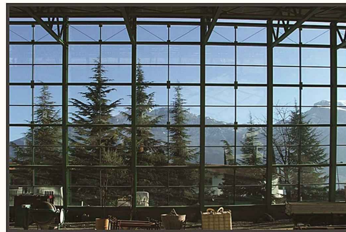
2000: Steel structure for Gimnasyum Limone del Garda, Brescia Our role: We were commissioned by the municipality to produce the architectural and structural design of a public gym in front of the lake. The structure is an asymmetric frame pinned at the base to minimize the flexure transmitted to the foundations.
